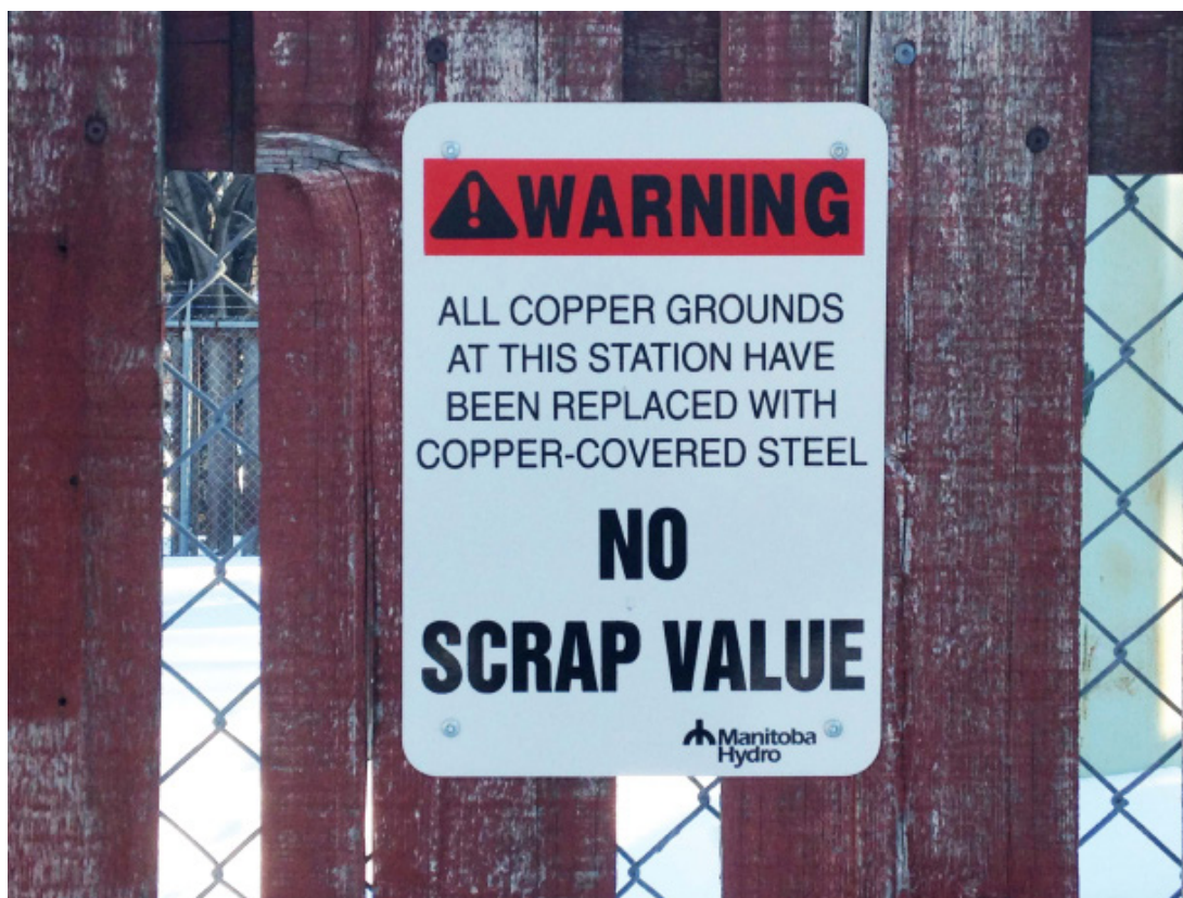
Figure 4: Signage at electrical substation
